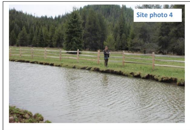
Repair site in Colby Meadow. Ditch plug 8 (foreground in site photo 3) was installed in the ditch to create wetland cells to reduce erosion, increase infiltration, and create wildlife habitat. Top two photos show prior condition; site photo 3 was taken the spring following completion of the ditch plug; site photo 4 taken the following fall, following installation of livestock exclusion fencing.
