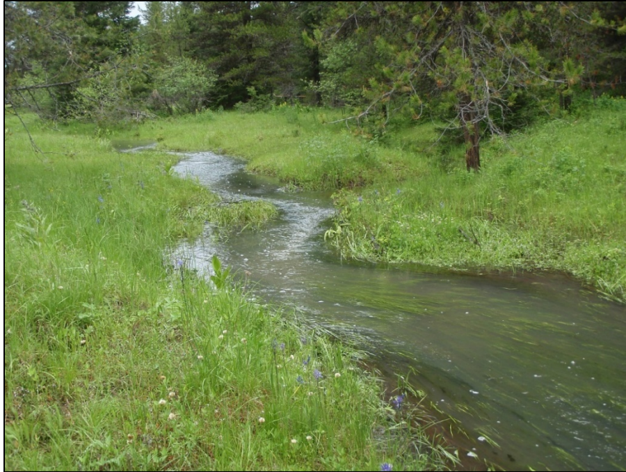
Figure 11. Corral Creek in Colby Meadow, June 10, 2010, 1-year post-construction. Corral Creek with flow following flow diversion from incised ditch and into historic channel alignment.
